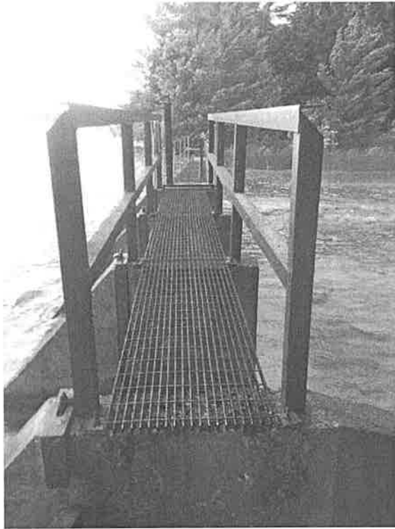
Structure from Right Bank
