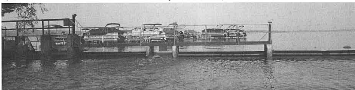
Figure 1.2.1. Image of the 2015 outlet control structure looking toward Higgins Lake from the Cut River. The low flow structure is in the center of the picture.
