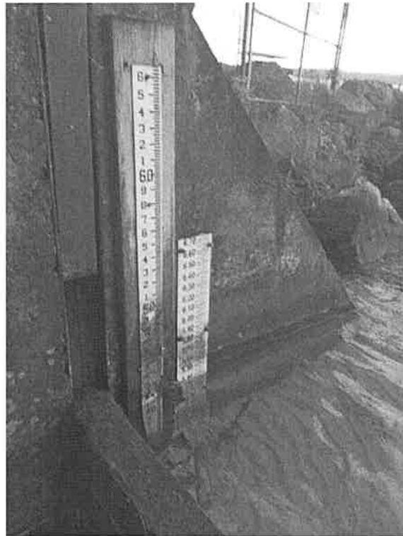
Right Abutment Wall, Staff Gage
