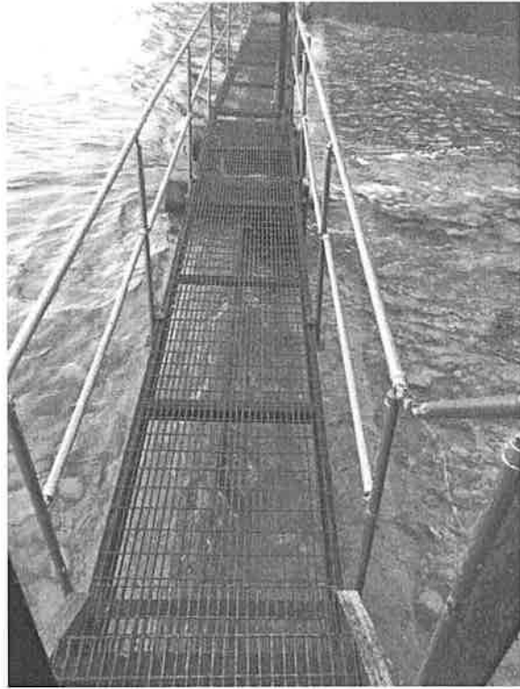
Left Catwalk with Newer Railing
