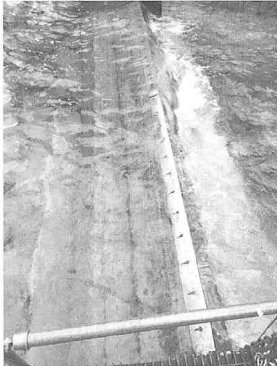
Typical Gated Bay (Note Gate Extension Plate on Right)
